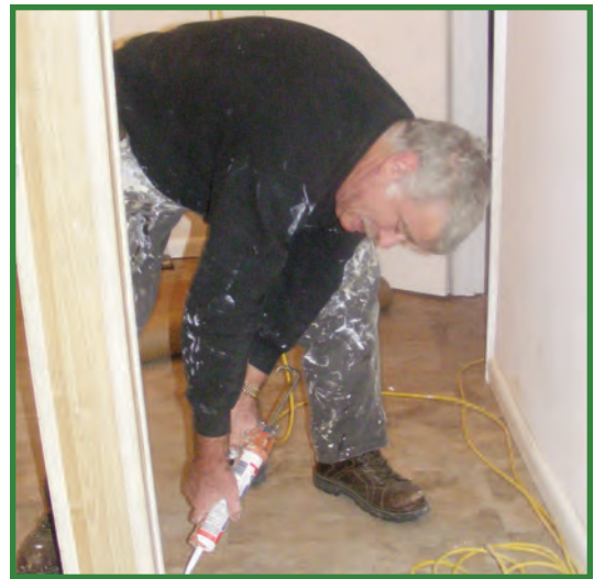
Walter Hall busily caulks the floor trim of the town home.
